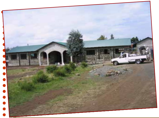
The Wendy Birrell Memorial Building nears completion at St Peters Huruma.
